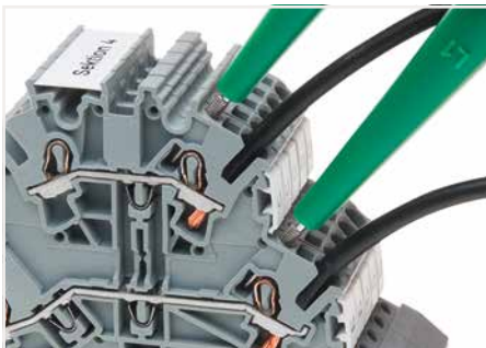
Testing with voltage tester.
